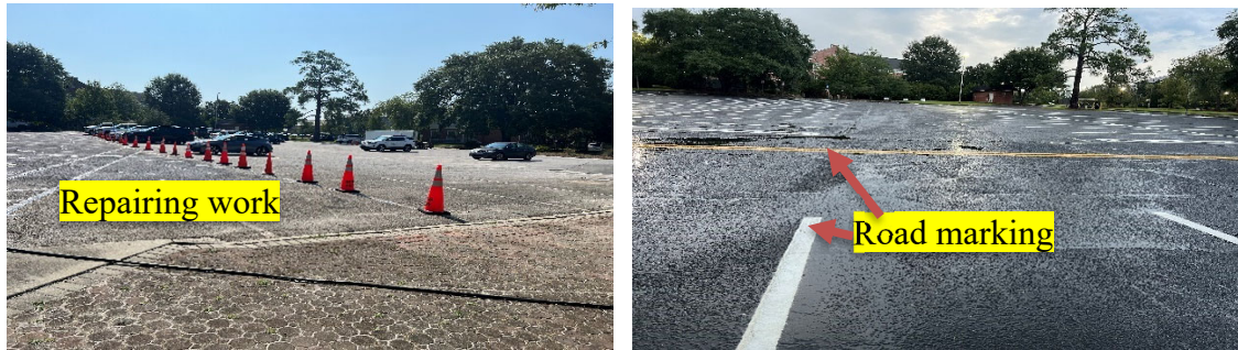
Figure 21. GSU Veazey Parking lot repairing work
