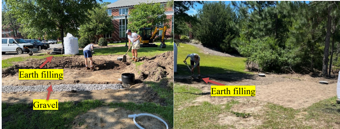
Figure 17. Earth Filing at Field Test Site
