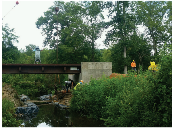
Figure 8. (Top) Culverts Forming Fish Passage Barrier at Pegamore Creek/Lee Road Crossing and (Bottom) Free-Span Bridge Installed at Pegamore Creek/Lee Road Crossing.
