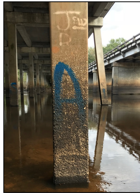
Figure 1: Bridge Site Columns
