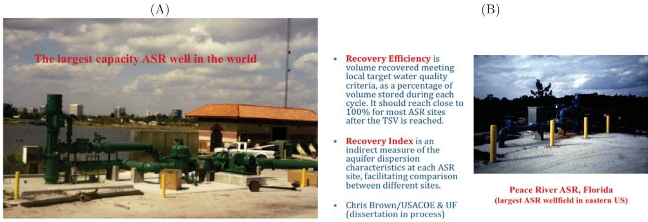
Figure 2: Photographs of: (A) West Palm Beach, Florida ASR well, described as the largest capacity ASR well in the world, equipped for 8 MGD capacity and abandoned because of recovery problems; and (B) Peace River, Florida ASR well, described as the largest ASR wellfield in the eastern US (from Pyne, 2004).
