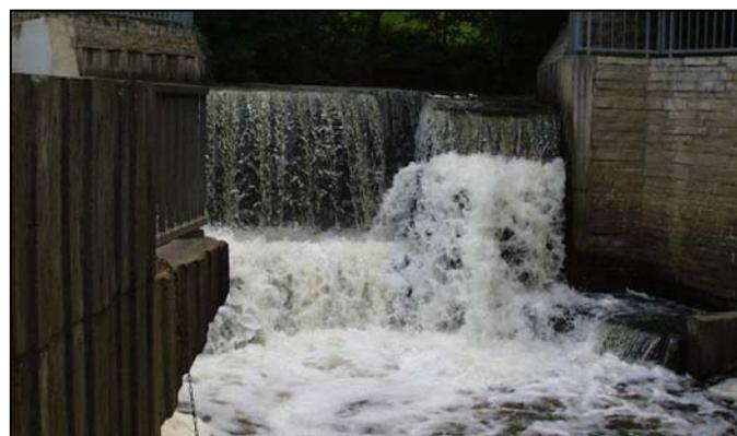
**Figure 3. Drop structure in Webber Park that disconnects Shingle Creek from the Mississippi River.**
