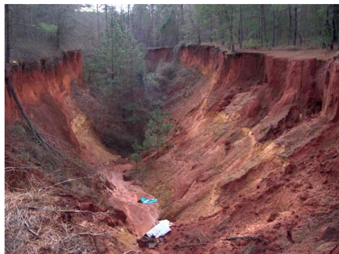
Figure-3 Extreme erosion and downcutting into soft Claiborne Group sandstone (lighter material) after breaching of the more resistant Altamaha sandstone (dark red sandstone on top), a road culvert concentrated storm runoff and caused the development of this canyon. Mass-wasting with down-dropped blocks of the Altamaha Formation occurs due to slope failure. Refrigerator at bottom of canyon for scale.
