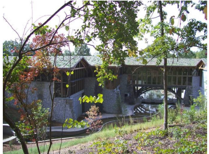
Cooling shoals water feature and newly planted green roof.
