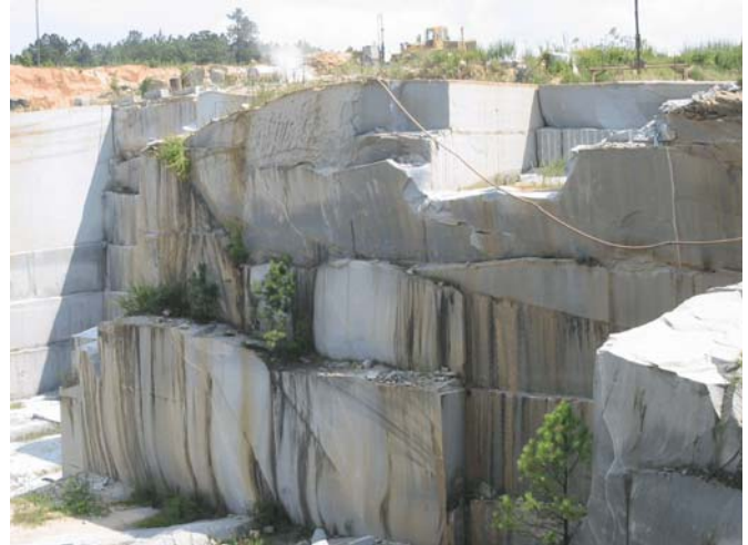
Figure 2. View of the south end of the Keystone Memorials Blue Quarry near Carlton, Georgia, showing water bearing fractures in one area as noted by evidence of wetting and the occurrence of trees and scrubs. Note the horizontal water-bearing fracture is connected to a steeply dipping fracture that extends upward to the surface.
