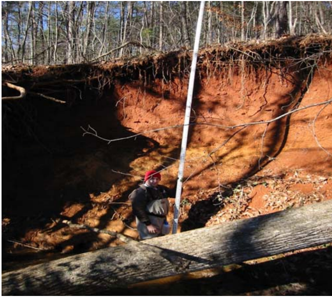
Figure 1. Severe Streambank Erosion In Butler Creek
