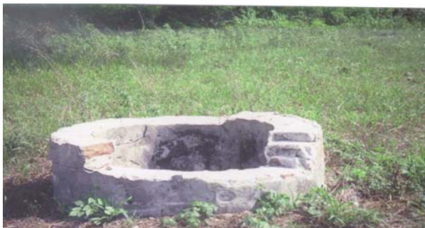
Figure 1. Abandoned hand dug well that was located at the roadside and identified for plugging.
