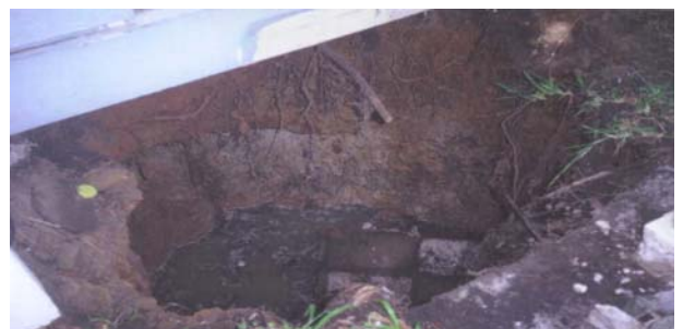
Figure 2. Abandoned well with foreign materials inside without casing at rear of house that was identified to be filled.
